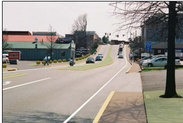
Figure T-3: Suburban-Style Complete Street Retrofit
