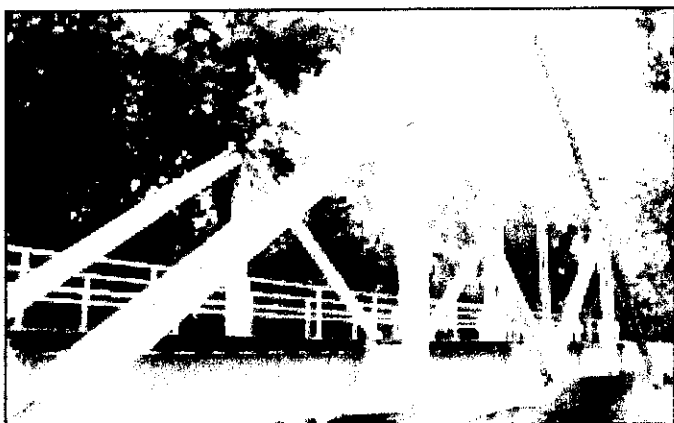
Under a Section 106 agreement, the U.S. Army Corps of Engineers dismantled and stored one of the Nation's last historic Waddell A-Truss bridges to save it from flood damage during construction of Smithville Lake in Missouri. Collaborative efforts led to its reconstruction in a local riverside park.
